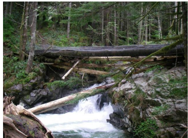
User-built structures such as this log bridge at Reiter Foothills Forest with chicken wire nailed to the top present risks to public safety and potential liability issues for DNR.
